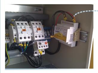
The Netbiter is connected to the control panel using the internal Modbus network.
