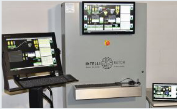
Egan Company designed and built batching control systems for seven (7) different production lines at a new TCC Materials plant. Electrical controls, air lines, plumbing, heating, temperature controls, ventilation and dust collection were installed on the production lines. Office and laboratory spaces were also fitted with electrical and HVAC systems.
