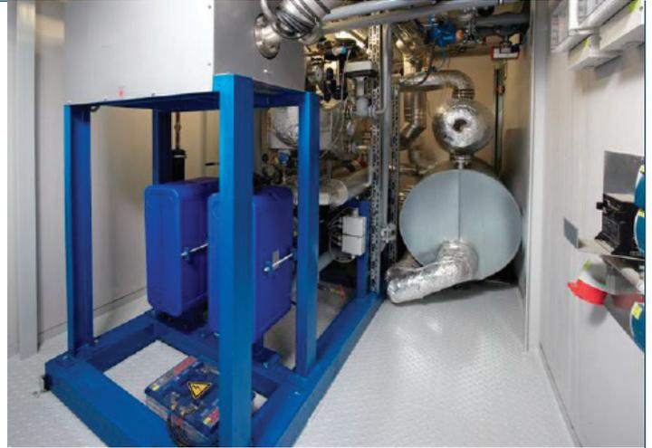
ORC (Organic Rankine Cycle) systems generate energy from process heat originating from industries, waste disposal sites and also as a by-products from electricity generation. Also here, remote maintenance is provided by Ewon.
